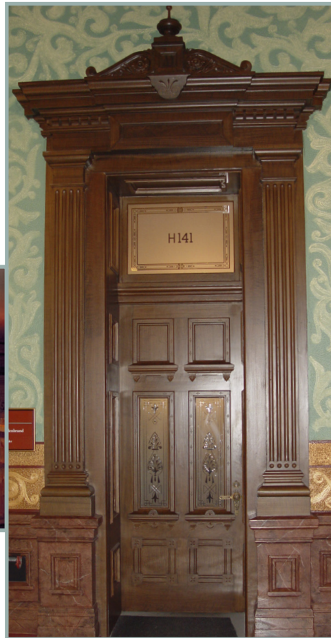
The Capitol's traditional woodgraining recipe calls for oil paints, umber pigment, and stale beer, which serves as the binder.
