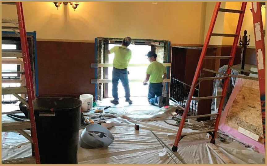
Installing a new window in S402.
