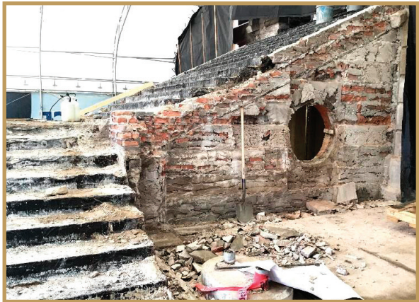
The old brick understructure of the south exterior stairs.
