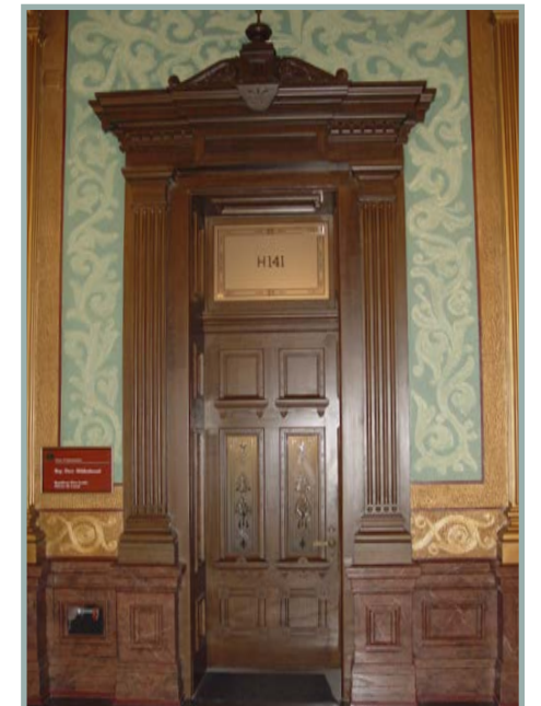
The Capitol's traditional woodgraining recipe calls for oil paints, umber pigment, and stale beer, which serves as the binder.
