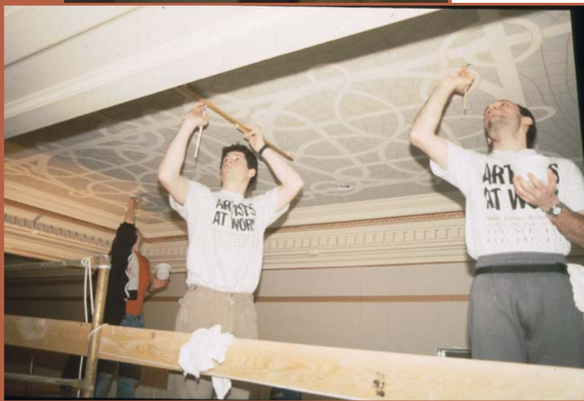
Decorative painters from across the country and around the world labored to recreate acres of decorative motifs. Much of the Capitol's most elaborate art can be found on or near the ceilings, which emphasizes the impressive height of the rooms.
